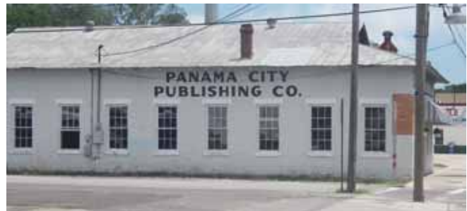
Panama City Publishing Co. Bldg, On Beck Avenue, Center of the Waterfront Commercial Area
