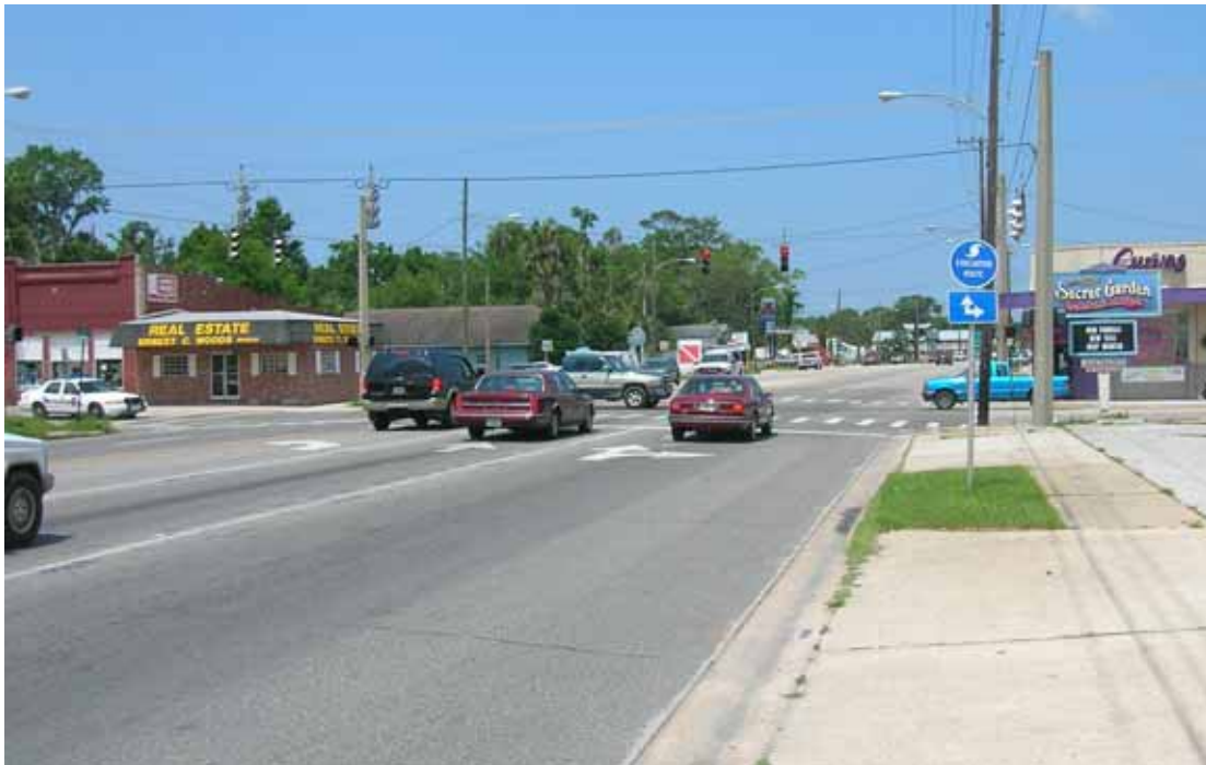
State Highway 19 is designed for dangerous high speed vehicular traffic and limits safe pedestrian walkability and the commercial viability of the historic downtown.
