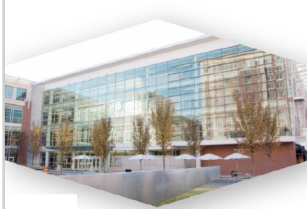
Energy Innovation Center Pittsburgh, PA
