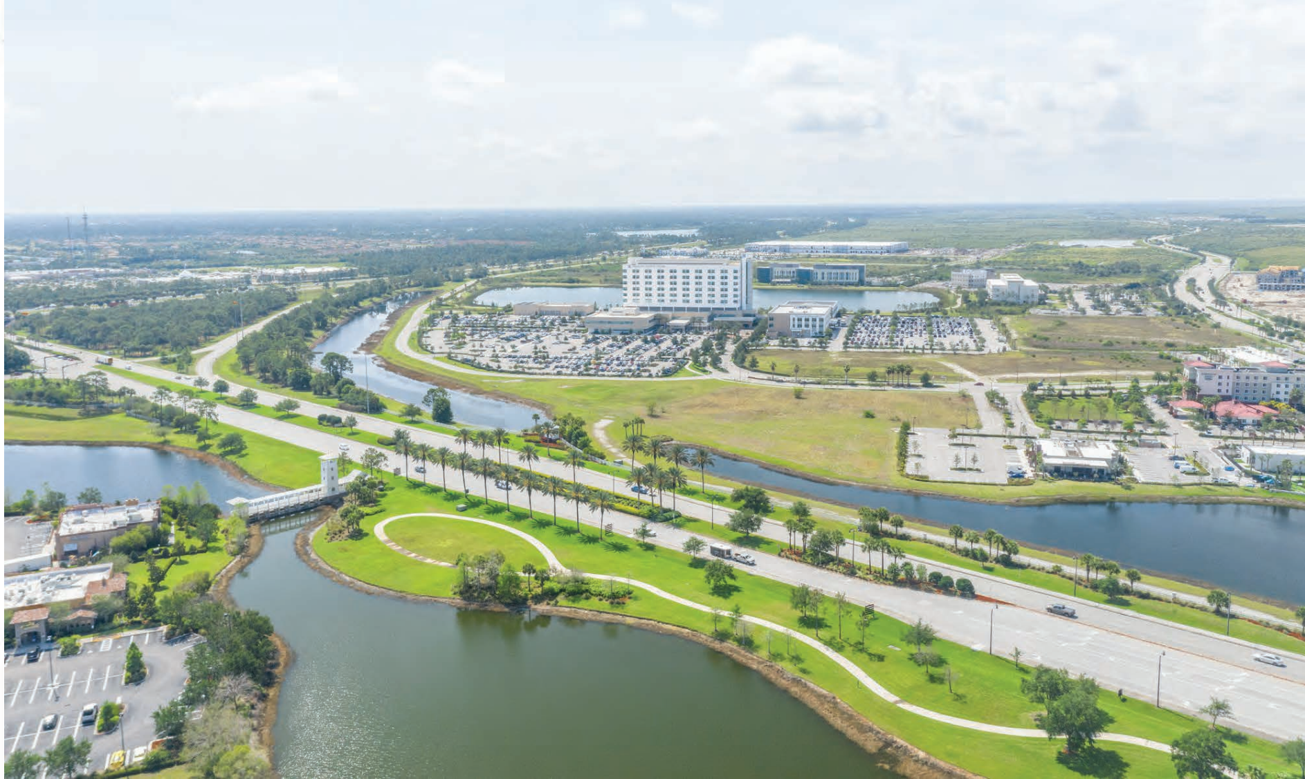
Photo 1, Tradition Center of Innovation (view from north to south)
