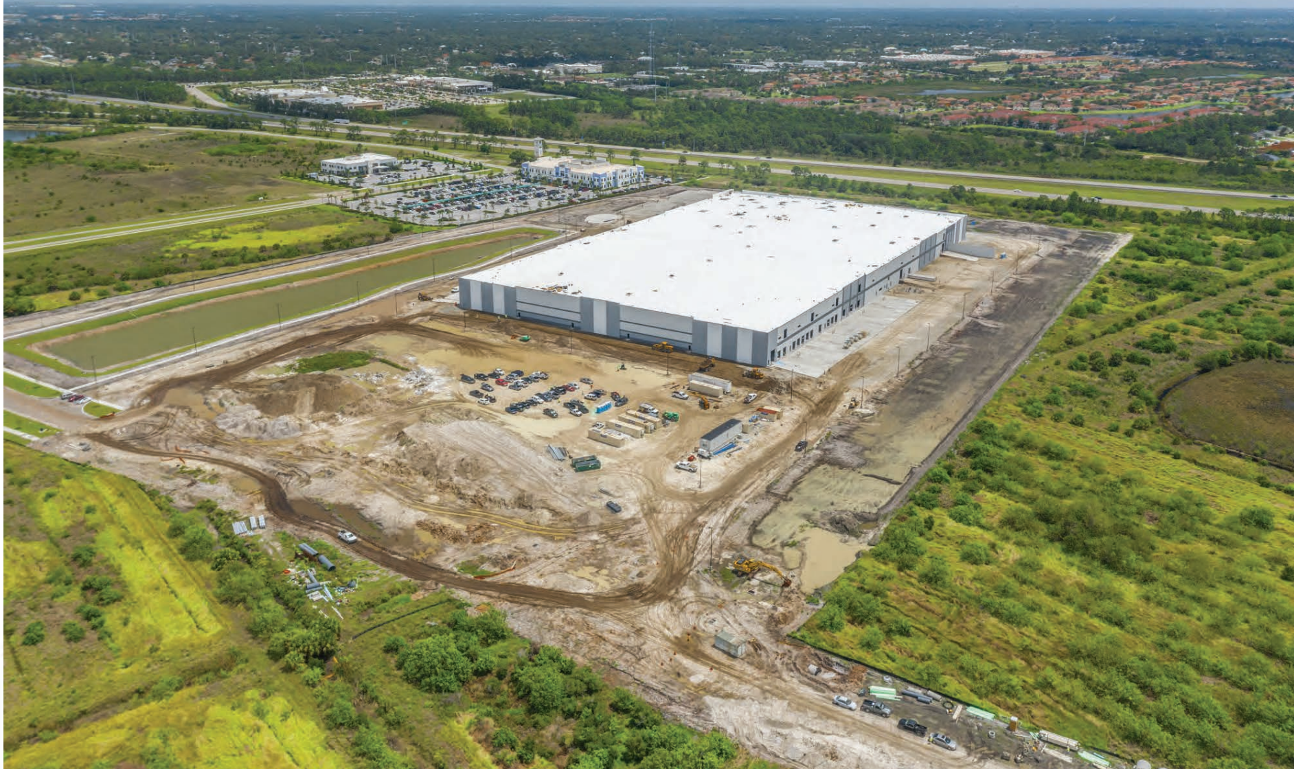
Photo 6, City Electric Supply/TAMCO (view from southwest to northeast)
