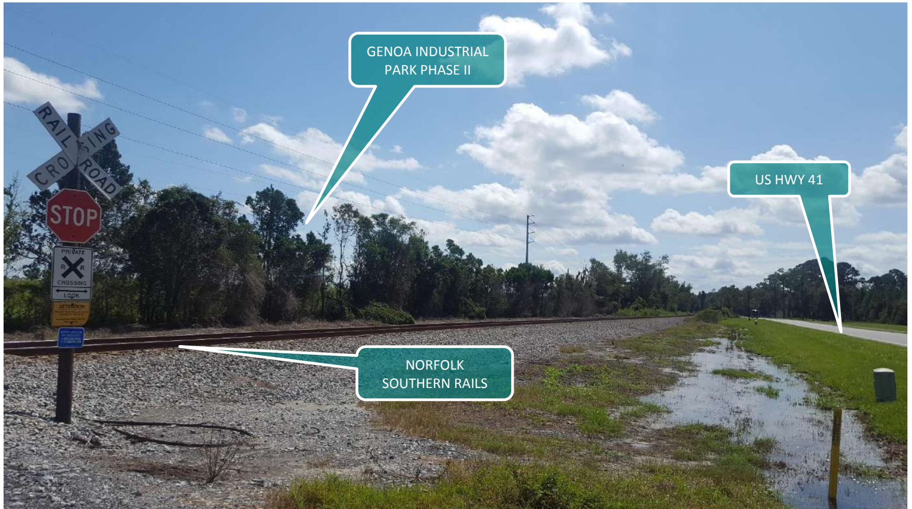
Image showing the entrance crossing to the project site and conditions after Hurricane Irma.
