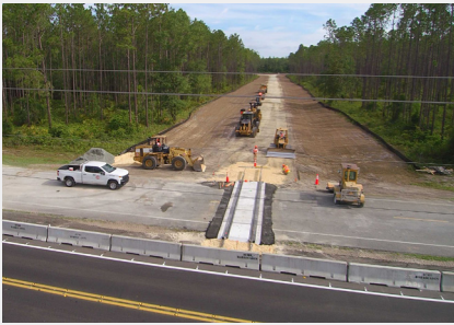
Construction of the Railroad Spur.
