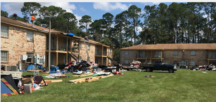
Clean up from the flooding in the first floor units.
