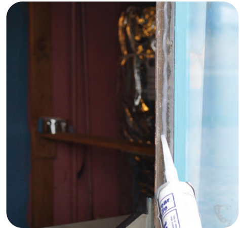
4. Run interior bead of caulk
