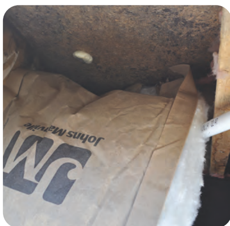
3. Batt vapor retarder faces warm side of floor
