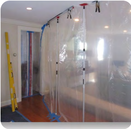
1. Protect work area from debris and dust
