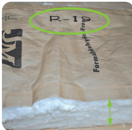
2. Insulation R-value matches work order
