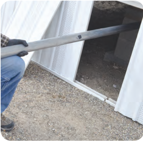
5. Fill entire belly cavity to prescribed R-value
