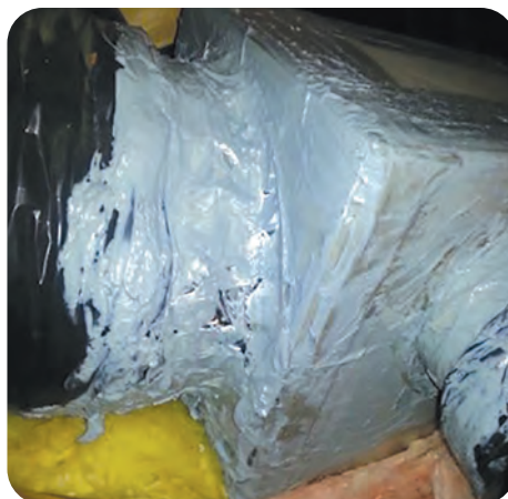
4. Seal new joints
