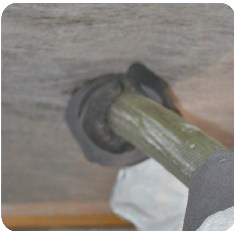
13. Loose fill netting to required density
