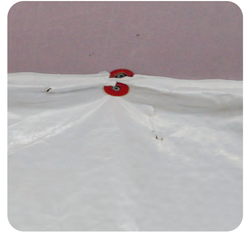
3. Seal seams of belly wrap
