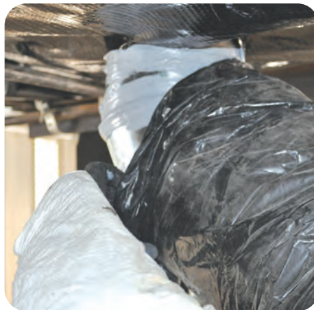
2. Pull insulation over hard connections as needed
