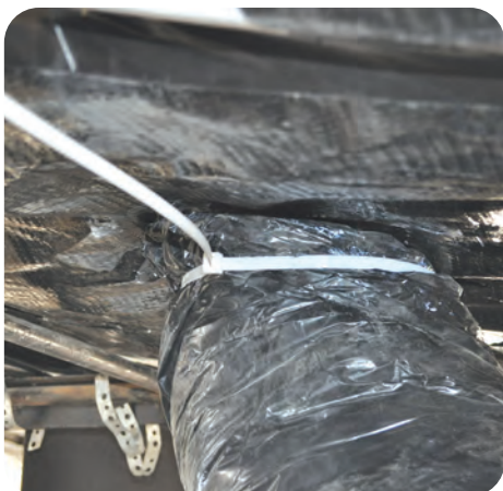
3. Secure vapor retarder layer at boots
