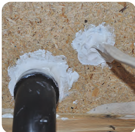
1. Ensure air sealing is complete
