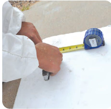
2. Cut blocking material to fit
