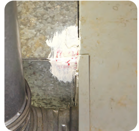
B-3. Apply mastic over the tape
