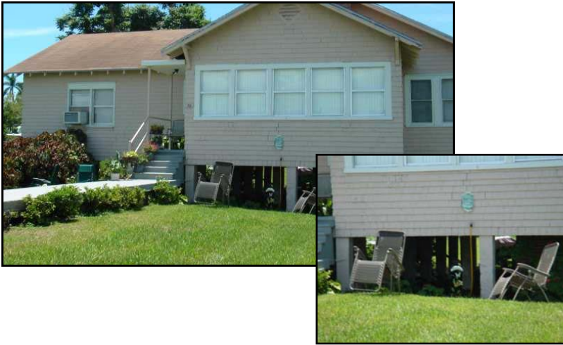
Figure 4 shows a house in the Glades Communities, with an exposed foundation due to the impacts of land subsidence. The second overlay picture shows a close up of the foundation of the house. Source: CSA, 2006.
