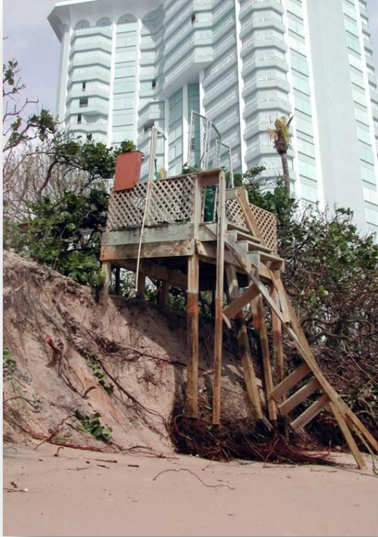
Photo (above): Damage to the Singer Island shoreline in Palm Beach County, Florida after Hurricane Frances. Courtesy of the Department of Environmental Resources Management for Palm Beach County (October 2004).
