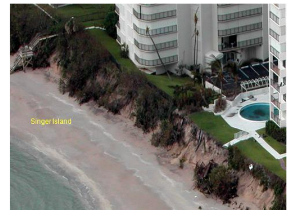
Photo (above): Damage to the Singer Island shoreline in Palm Beach County, Florida after Hurricane Frances. Courtesy of the Department of Environmental Resources Management for Palm Beach County. (October, 2004).
