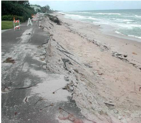
Photos (above): Road erosion on Old South Ocean Boulevard due to Hurricane Frances in 2004 in Palm Beach County, Florida (before and after). Courtesy of the Palm Beach County Department of Environmental Resources Management (2004).
