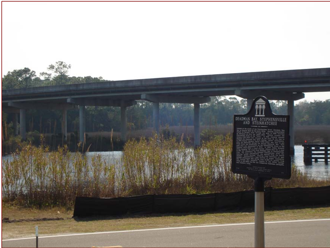
Steinhatchee Bridge and view of Deadman Bay
