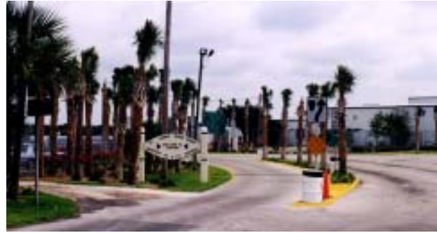
Recent landscape improvements at the FDOT ferry slips have significantly improved the visual appearance of both the Mayport Village and the Ft. George landings.
