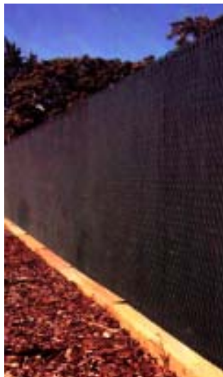
Where chain link fencing cannot be avoided, attractive colored slats or vinyl coating should be used
