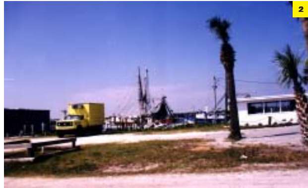
Shallow lot with building is not suitable for new construction.
