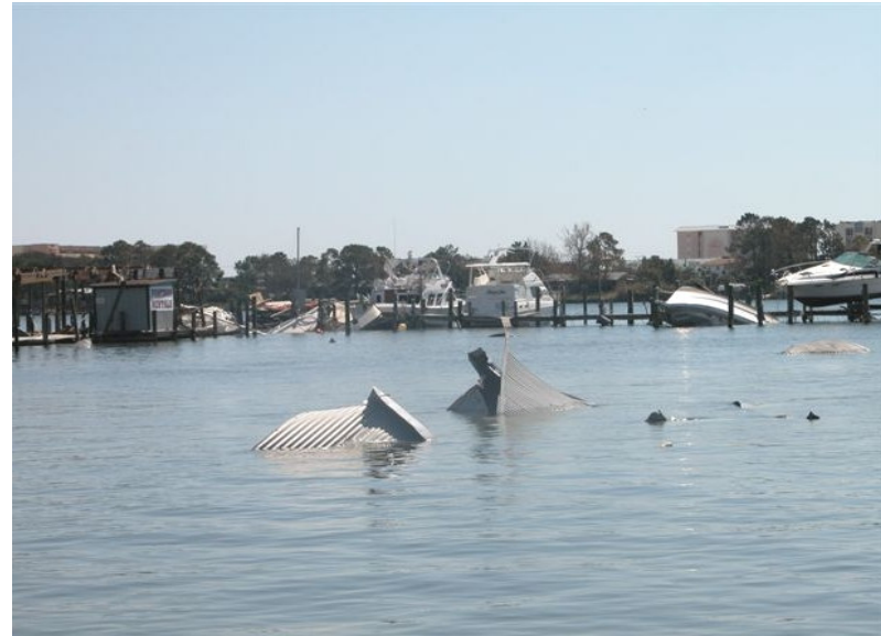
Hurricane Ivan caused extensive damage along the Santa Rosa Sound waterfront in October 2004. Here, the remains of sheet-metal roofing from a marina rest on the shallow bottom.
