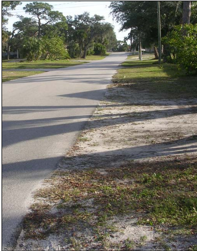
Figure 6 On-Street Public Parking (Block 1, Creel Avenue)
