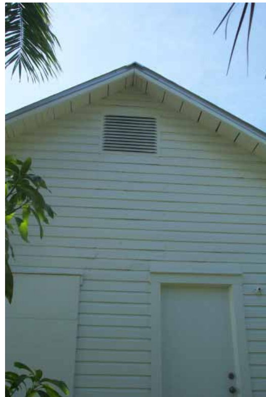
34: North Wall Detail
