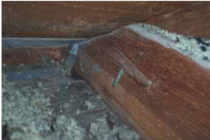
107: Joist End at Exterior Wall
