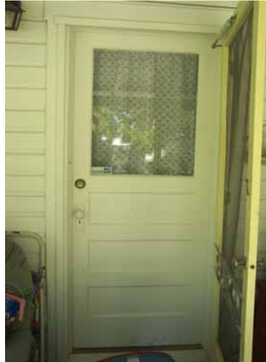
36: Door at West Elevation
