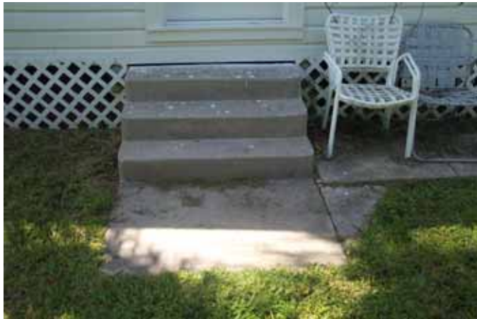
35: Steps at North Elevation
