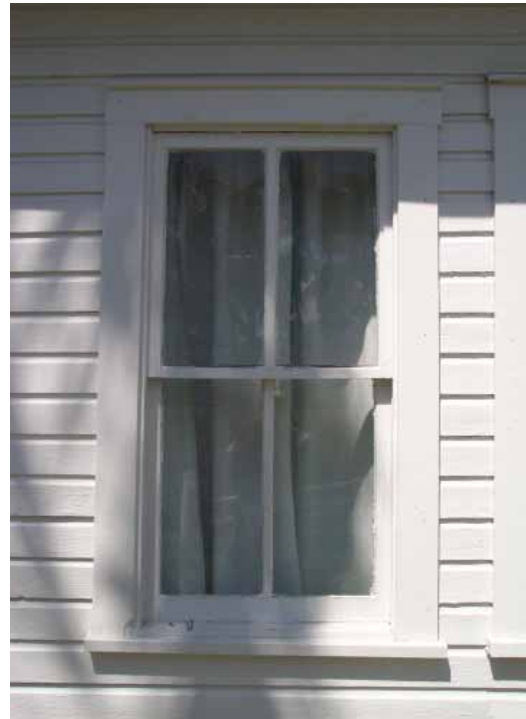
28: Window Detail - East Elevation
