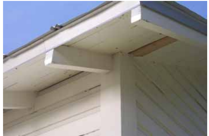
30: Roof Framing Detail - Northeast Corner
