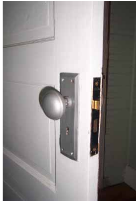
90: Door Lock Detail - Mortise Lock
