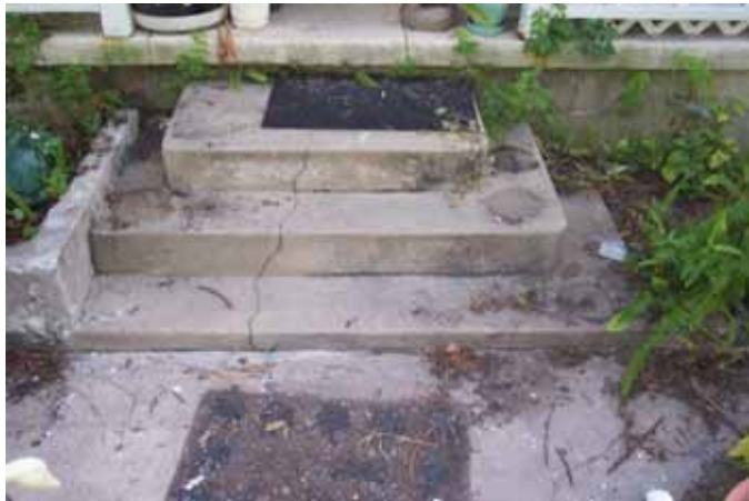
39: Steps at West Elevation
