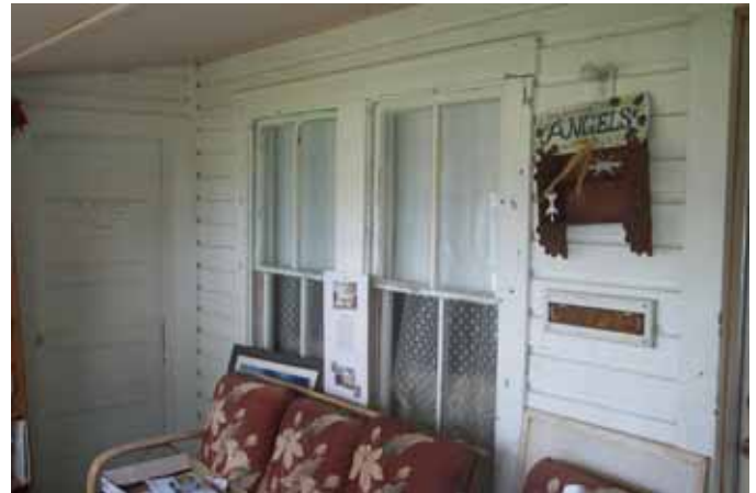
96: Front Porch - Partial Wall at West End
