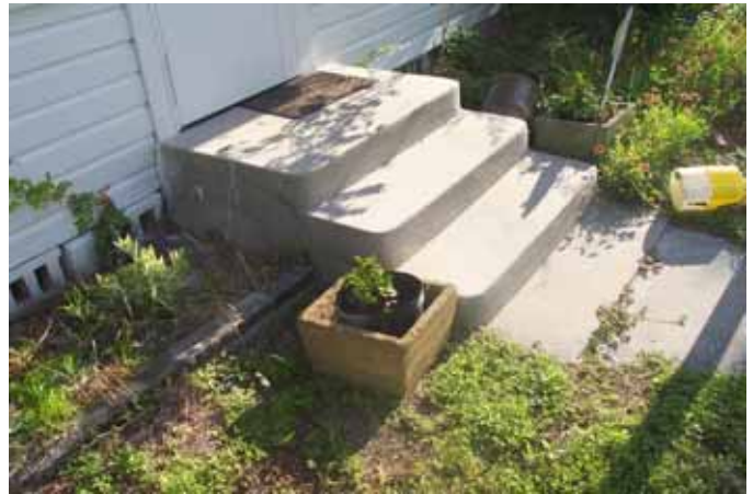
38: Steps at South Elevation
