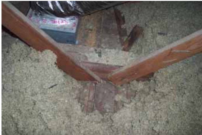
101: Detail of Ceiling Joist bracing over Control Wall
