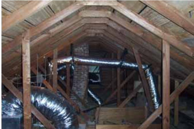
97: Attic looking North
