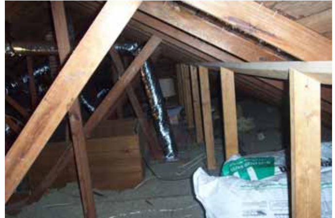
98: Attic looking South - Support Detail
