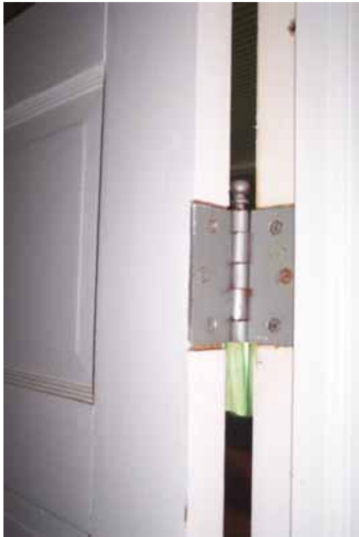
89: Door Hinge Detail - Ball Tipped Hinge
