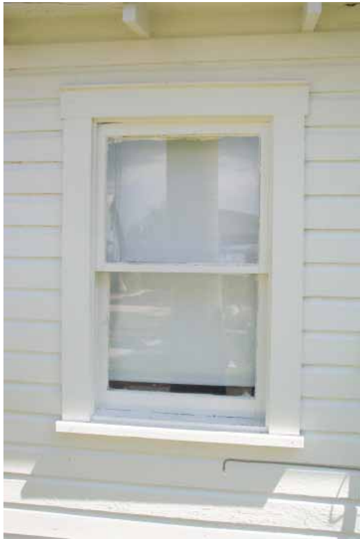
25: Window Detail - South Elevation
