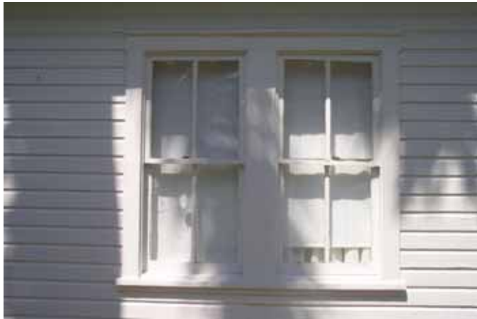
29: Window Detail - East Elevation
