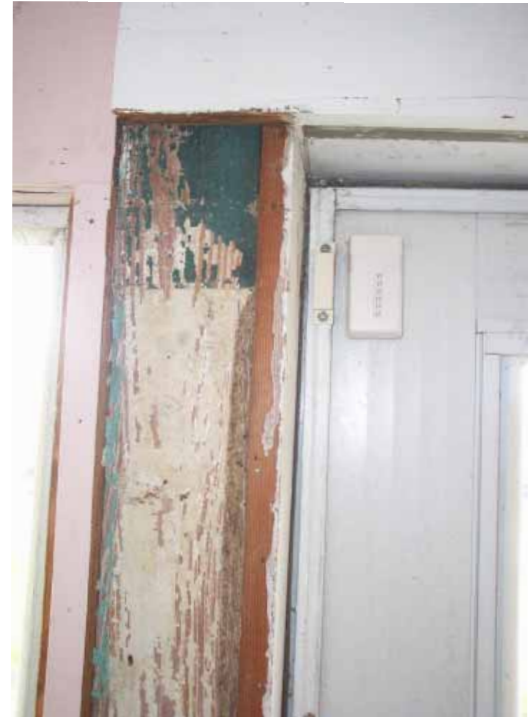
92: Detail at Original Chamfered Porch Column
