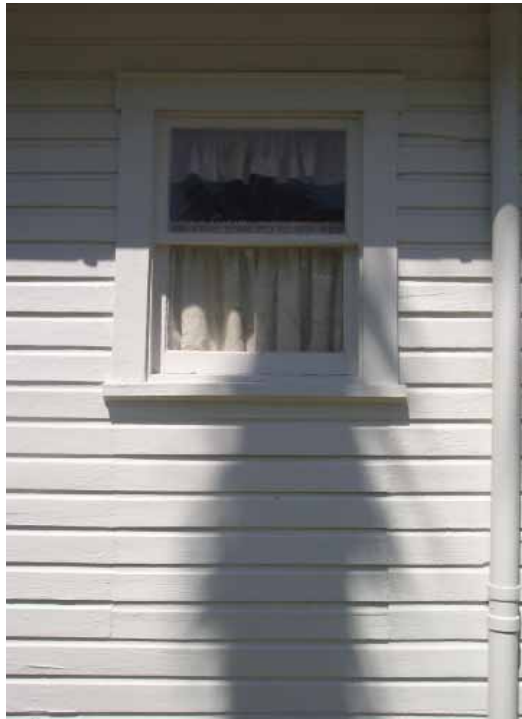
27: Window Detail - East Elevation
