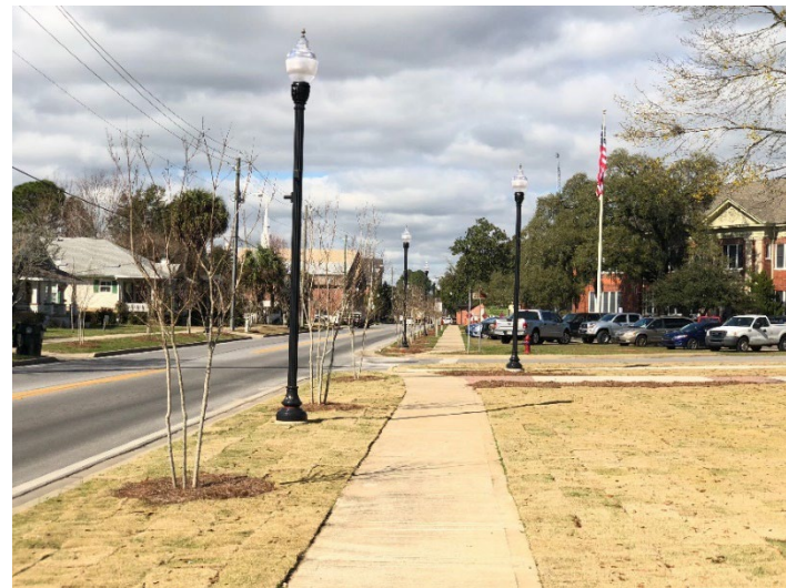
Commercial Revitalization – Milton: New underground utilities, sidewalks and lighting.
