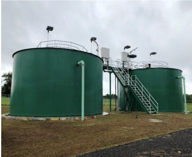
Neighborhood Revitalization – Greenville: Construction of a new wastewater treatment plant.
