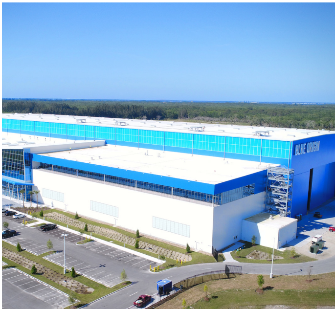
Blue Origin's New Glenn Orbital Launch vehicle program launch, manufacturing and support facility in Florida.
