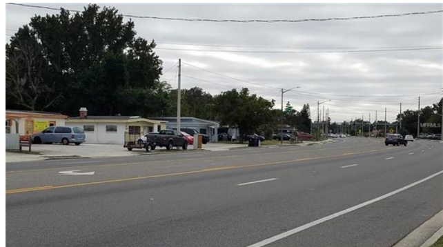
Figure 1: The existing built environment on North Pine Hills Road consists of 1950s and 60s ranch style homes that have been repurposed for professional office use. Many are in decline and dilapidated.
