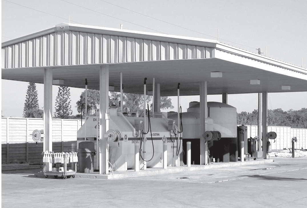
Figure 4.10. This wash pad and fuel island complex helps to prevent problems by containment and recycling.
