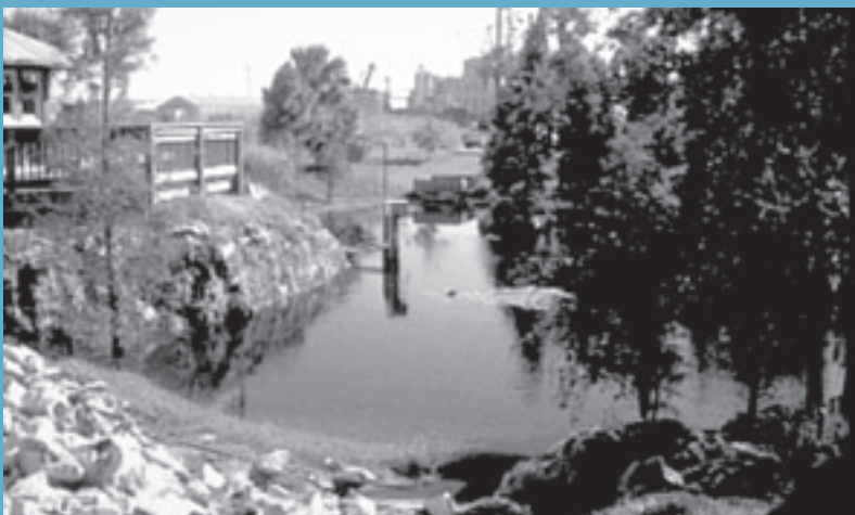
Figure 3.8. An integrated stormwater treatment train, including a wet detention pond, were used at the Florida Aquarium.
