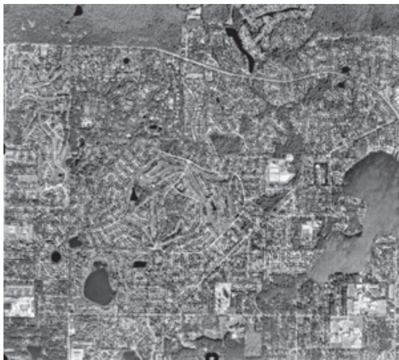
Figure 2.1. This aerial of Seminole and Orange counties shows Wekiwa Springs and State Park to the north and extensive development to the south within the springshed. Sand Lake and Lake Brantley can be seen along with golf courses and residential road networks.
