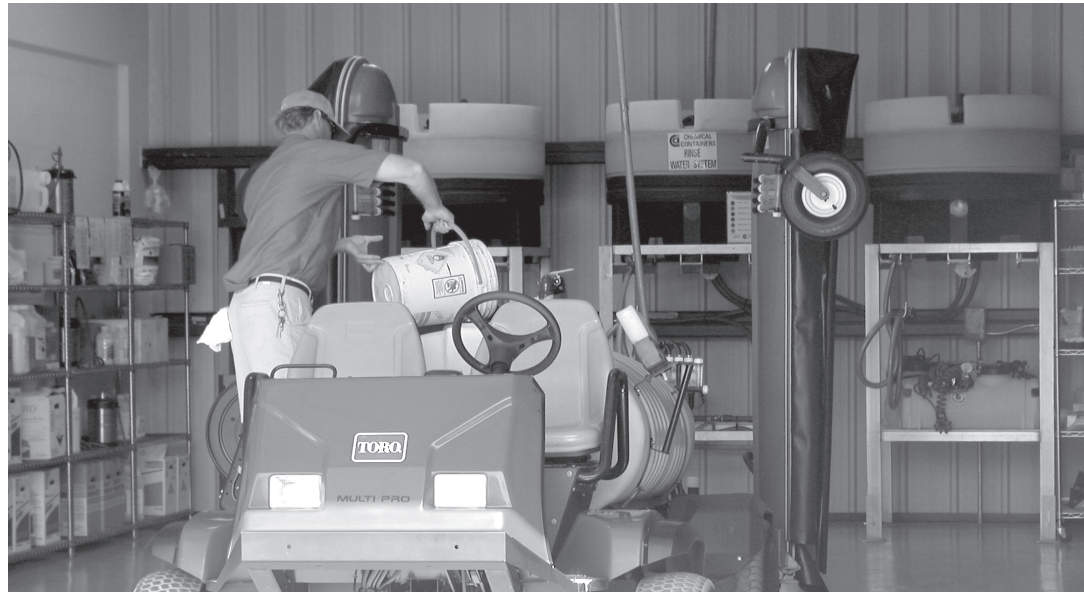
Figure 4.9. This pesticide storage, mixing and loading facility helps to prevent environmental problems by containment and recycling of rinsate water.
