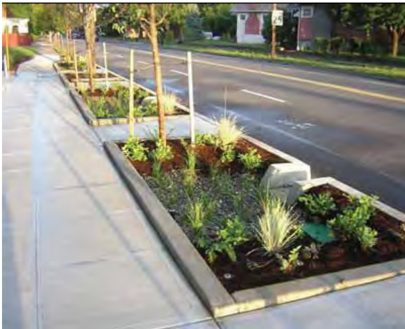
Figure 3-6. Street runoff is directed to landscaped bioswales for filtration and treatment. Where curbs are installed, curb cuts allow water to flow into the bioswale, which also provides street landscaping.
