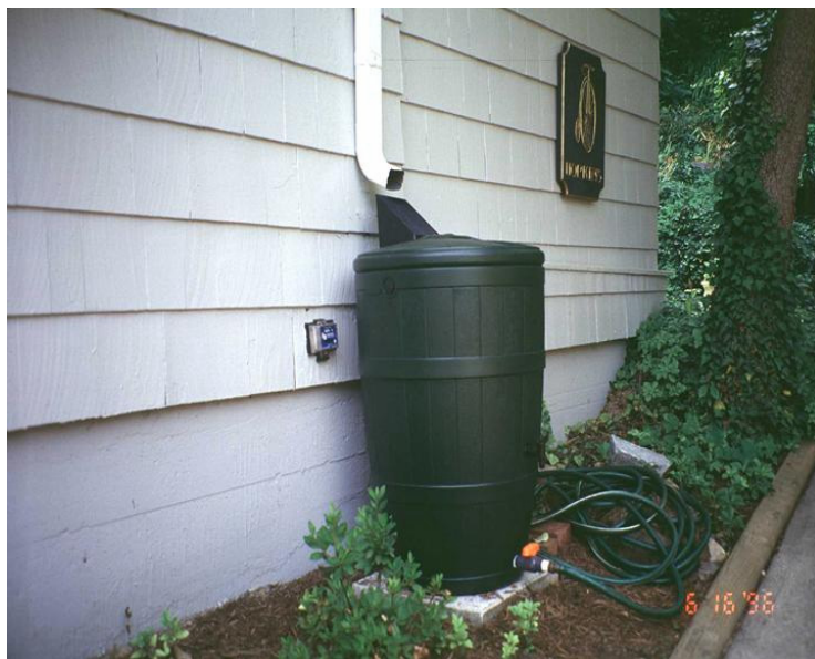
Figure 3-8. An example of runoff to a rain barrel. Source: Marty Wanielista, Stormwater Management Academy, University of Central Florida
