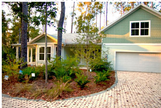
Figure 3-9. Permeable pavement increases recharge and reduces runoff. When combined with drought tolerant vegetation, stormwater is appropriately managed.
