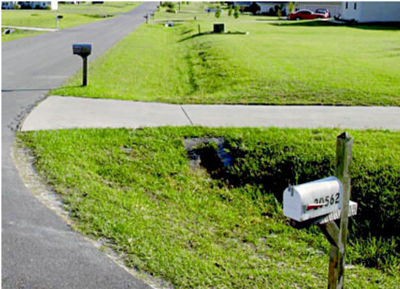
Figure 3-5. Swales are one means of managing stormwater runoff and ensuring recharge along residential streets. Swales are preferred over a curb and gutter design in many situations.
