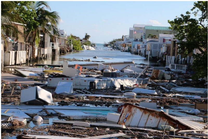
Debris-filled residential canal – Marathon (Source: B. Powell)
